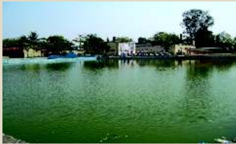
Pond Built in Shelgaon Gauri GP
